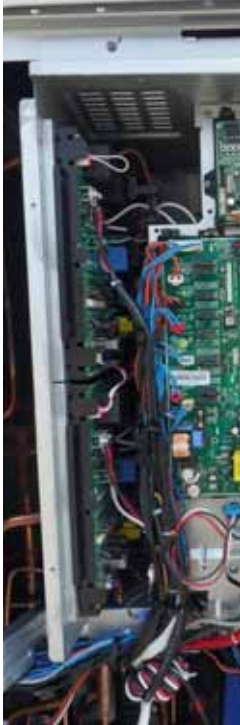
► Comp Wire fix by Holder Wire.
